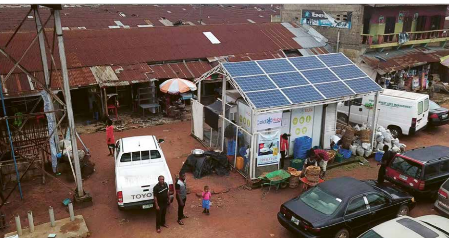
One of ColdHubs' solar-powered cold rooms in Nigeria
